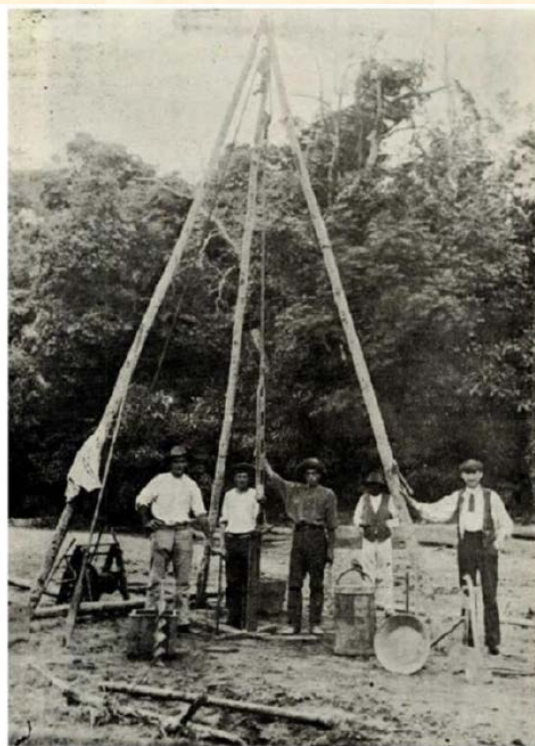
BORING FOR TIN ON THE ROMEO COMPANY AND CARSON DREDGING CLAIMS.
