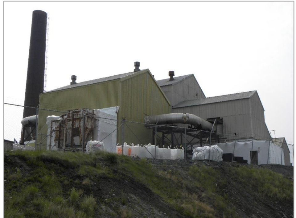
Roaster complex being dismantled (photo by John Sandlos)
