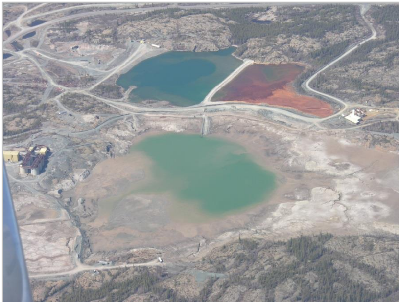
Giant Mine water treatment ponds (KOR)
